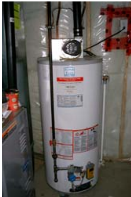
Checking for correct manifold gas pressure
