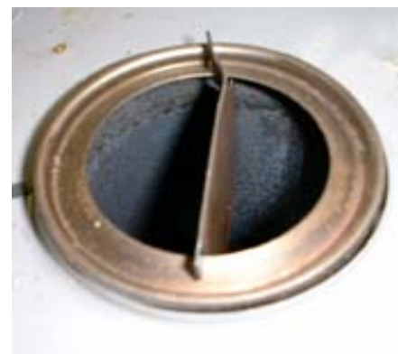
Correct Baffle positioning
