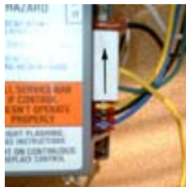
Sliding cover up to obtain voltage readings
