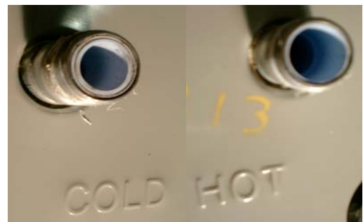
Cold and hot water inlets. Double lining on cold indicating presence of dip tub
