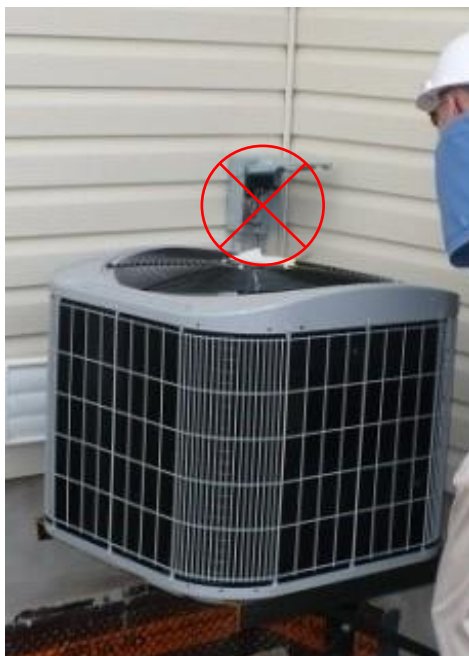
Photo 4 – 1 metre of working space required
