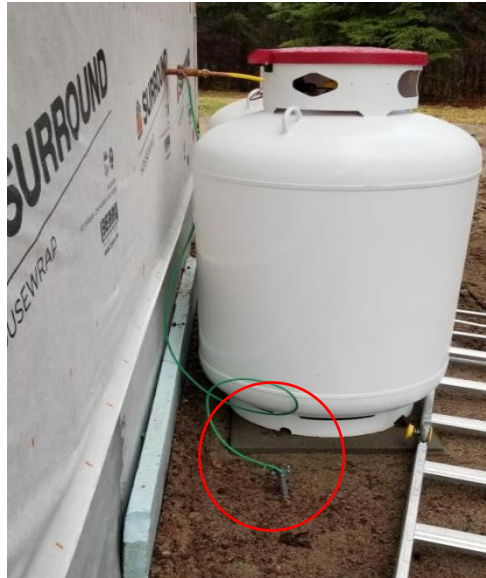
Diagram 12 – LP line connected to separate grounding electrode is not permitted
