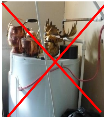
Photo 2 - NMSC not protected by location
