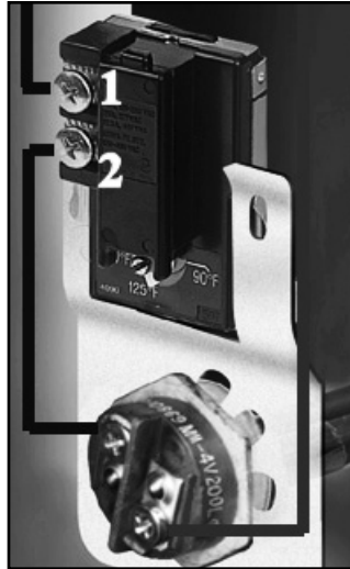
Figure 6 - Lower Thermostat & Heating Element Wiring
