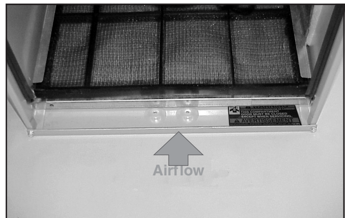
BOTTOM FILTER RACK INSTALLATION
